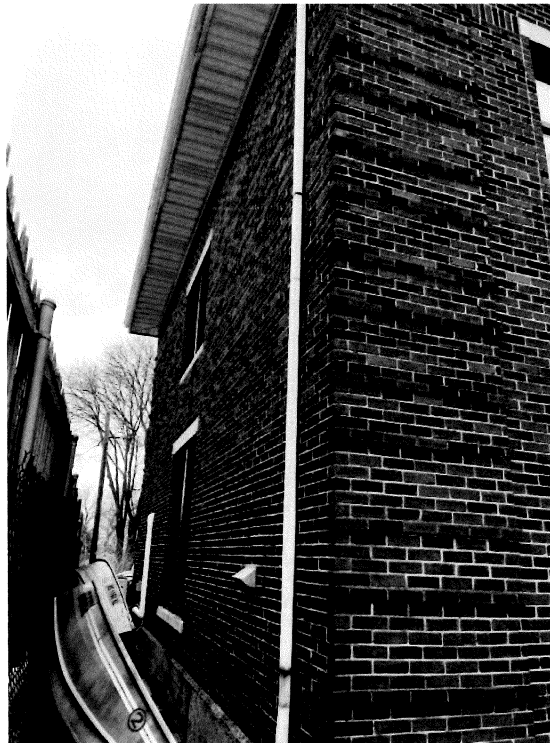
Building Rear View (West side)
