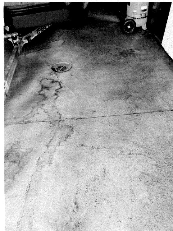
Floor Condition (Right Bay)
