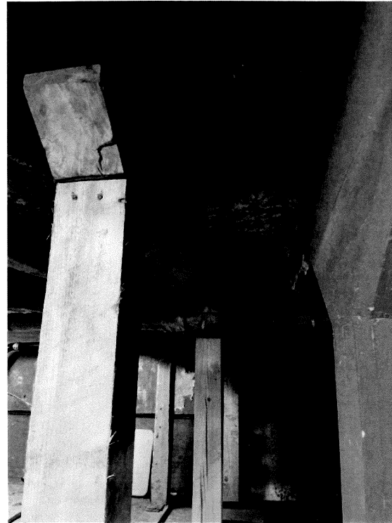
Floor Shoring (Left Bay)
